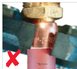
Jaw not square on the crimp ring
