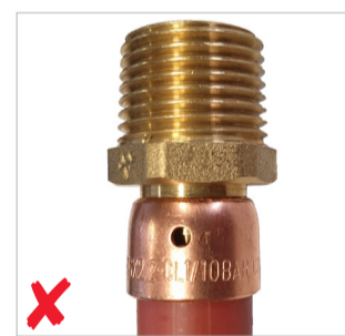
Witness hole not completely filled
