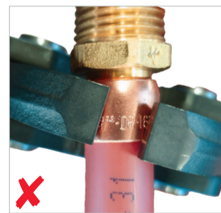
Jaw not square on the crimp ring
