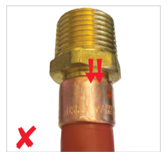
Fitting has been double crimped
