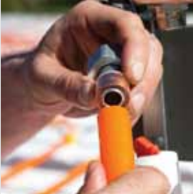
Step 14a. After deburring pipe, push fitting onto pipe
