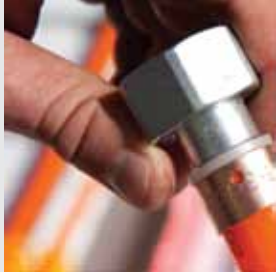
Step 14b. Slide fitting onto pipe, ensure the pipe is visible in viewing circle
